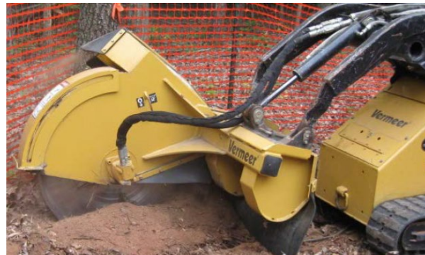
Figure 22. Root Cutting Machines Are Used to Sever Roots Interfering with Construction
