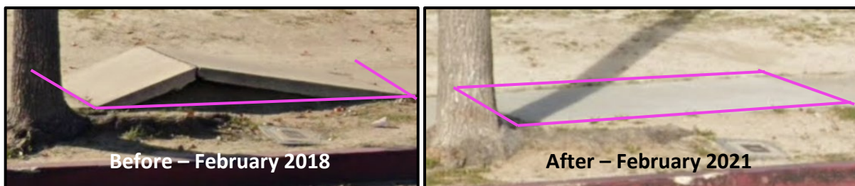
Figure 16. The Risk and Liability Mitigation Program Can Make Targeted Sidewalk Repairs
